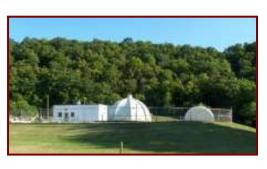
The Village's existing Waste Water Treatment Plant (WWTP) is located on the south side of State Highway 29. The WWTP has a design capacity of 115,000 gallons per day (gpd), with and average treatment of 40,000 to 70,000 gallons per day. The WWTP was last upgraded in 1984, but the plant still utilizes buildings/structures from 1949. The treatment plant is being replaced in 2010 as part of the recommendations set forth in the Spring Valley Facilities Plan.
